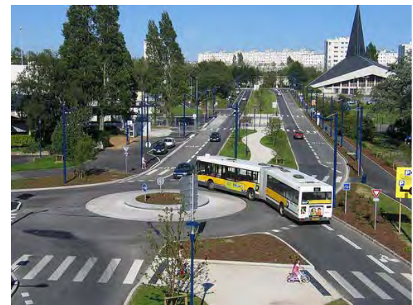
Figure 2 A multi-modal roundabout
